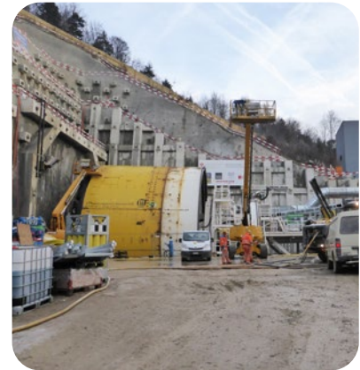
TBM on the south entrance of the tunnel
