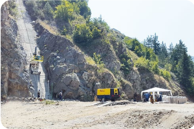
Grouting process of the left dam shore.
